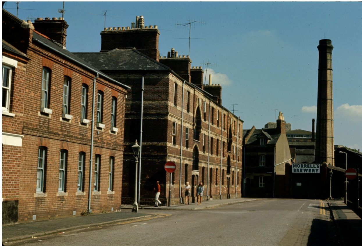
Figure 2. Christ Church Old Buildings in Osney Lane in 1971. The three storeyed tenement block of red and cream brick, designed by E. G. Bruton and built between 1866 and 1868, provided a mix of one, two and three bedroomed flats around a central drying ground. Beyond it, there is a glimpse of one of the Christ Church houses built in The Hamel in 1868 alongside Morrell's Brewery chimney.
