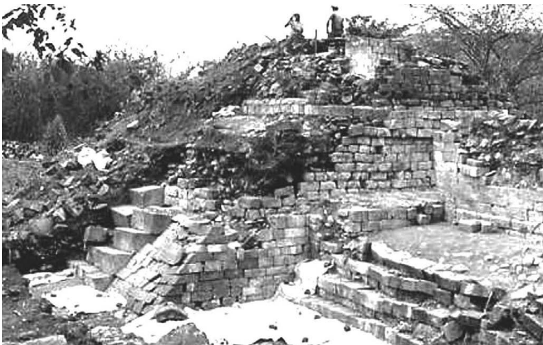
Figure 3-10. Southern half of Str. 22 excavated.
