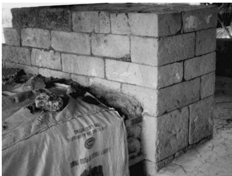
Figure 4-10. The south plinth of the bench and its joint with the Sky-band bench.
