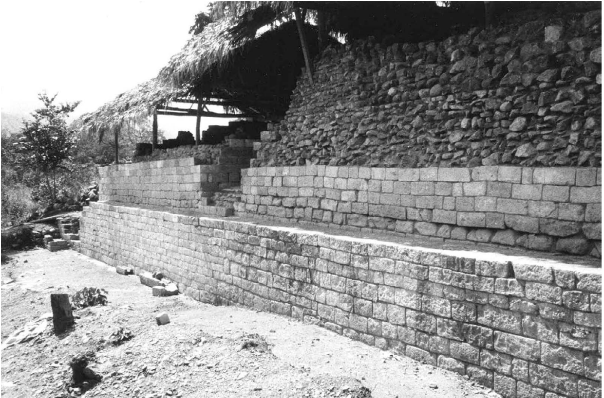
Figure 3-22. Rear retaining walls of Strs. 66C and 66S after restoration. The narrow corridor that separates the two buildings is visible on the second level. Note the absence of any visible seam in the lower wall.
