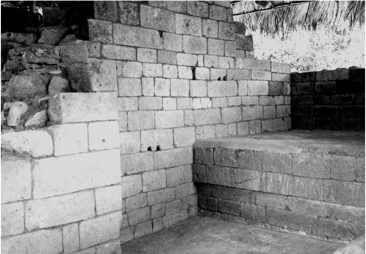
Figure 3-34. Interior of Room 2, Str. 66S. Jamb of main doorway on left, and cord-holders visible on north wall. Note the substantial but undecorated bench.
