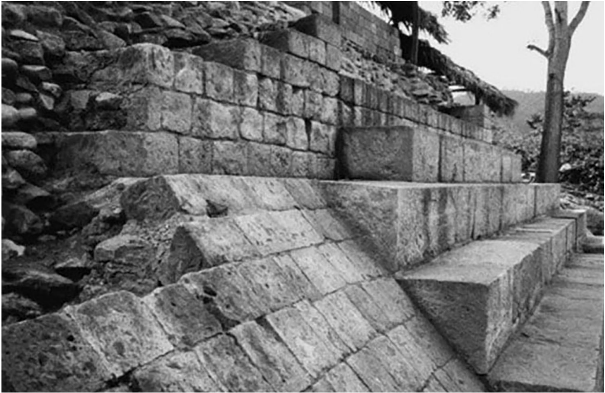
Figure 3-16. High-quality masonry on the taluds, stairway, and terrace-level walls. Front of Str. 66C.
