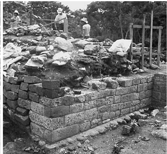
Figure 3-42. Northeast corner of Str. 66N after reconstruction. The wall of the North Platform is visible on the right.
