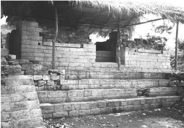
Figure 3-25. West façade of Str. 66S after restoration. The construction of the stairway is very different from that of Str. 66C. Fine quality masonry is evident both on the structure and the substructure.
