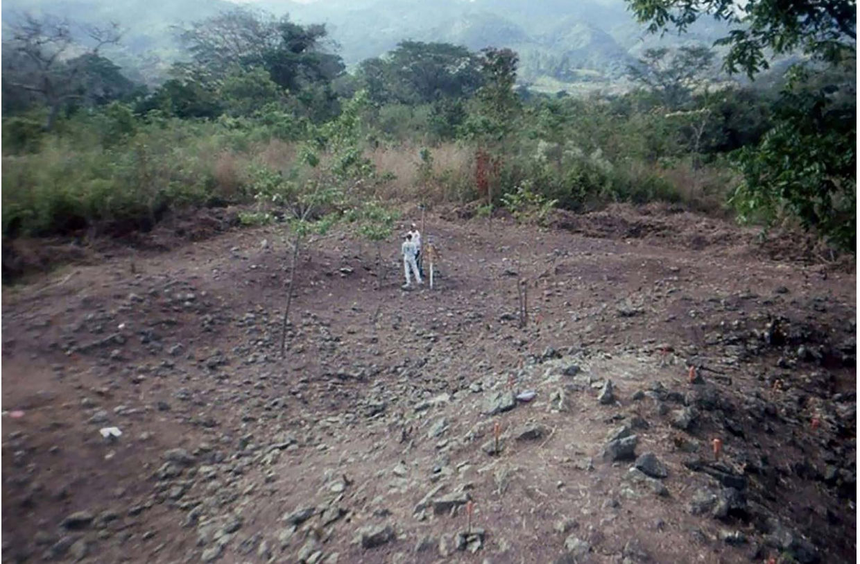
Figure 2-8. Clearing the site.
