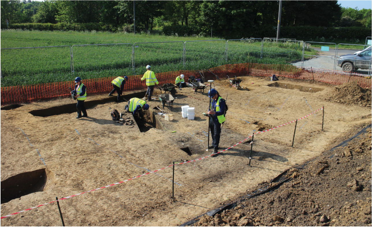
Plate 5: Excavating Area A, at the northern end of the Soff Lane diversion
