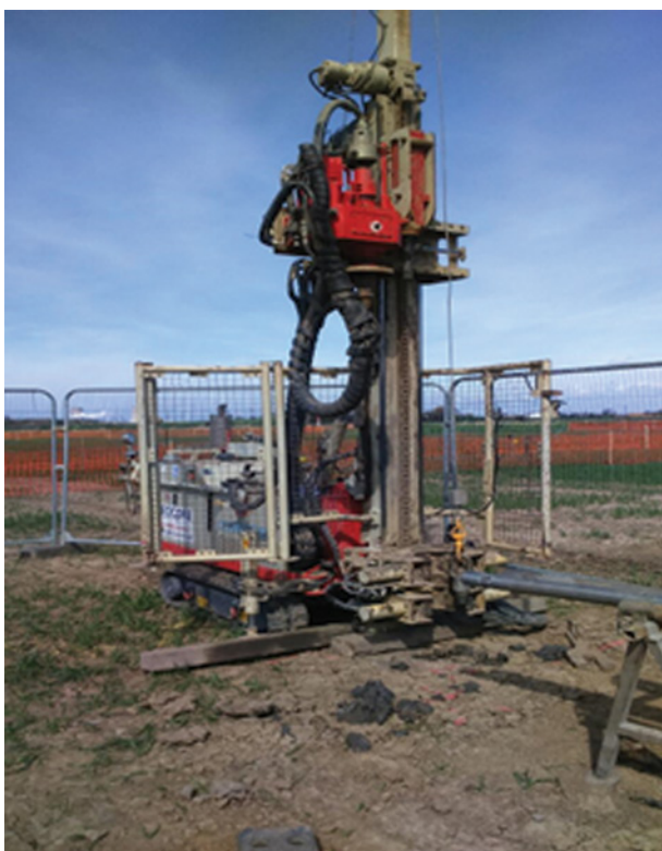
Plate 11: The tracked borehole rig extracting cores at Paull
